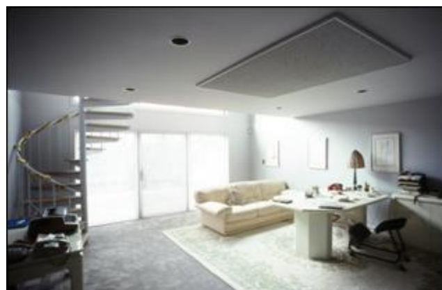
Figure 3 - Radiant ceiling panel in home office
